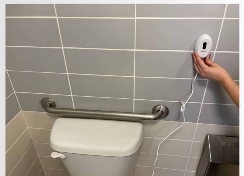
Hang The Sensor On The Wall And Make Sure Barrier-free 20cm Ahead
