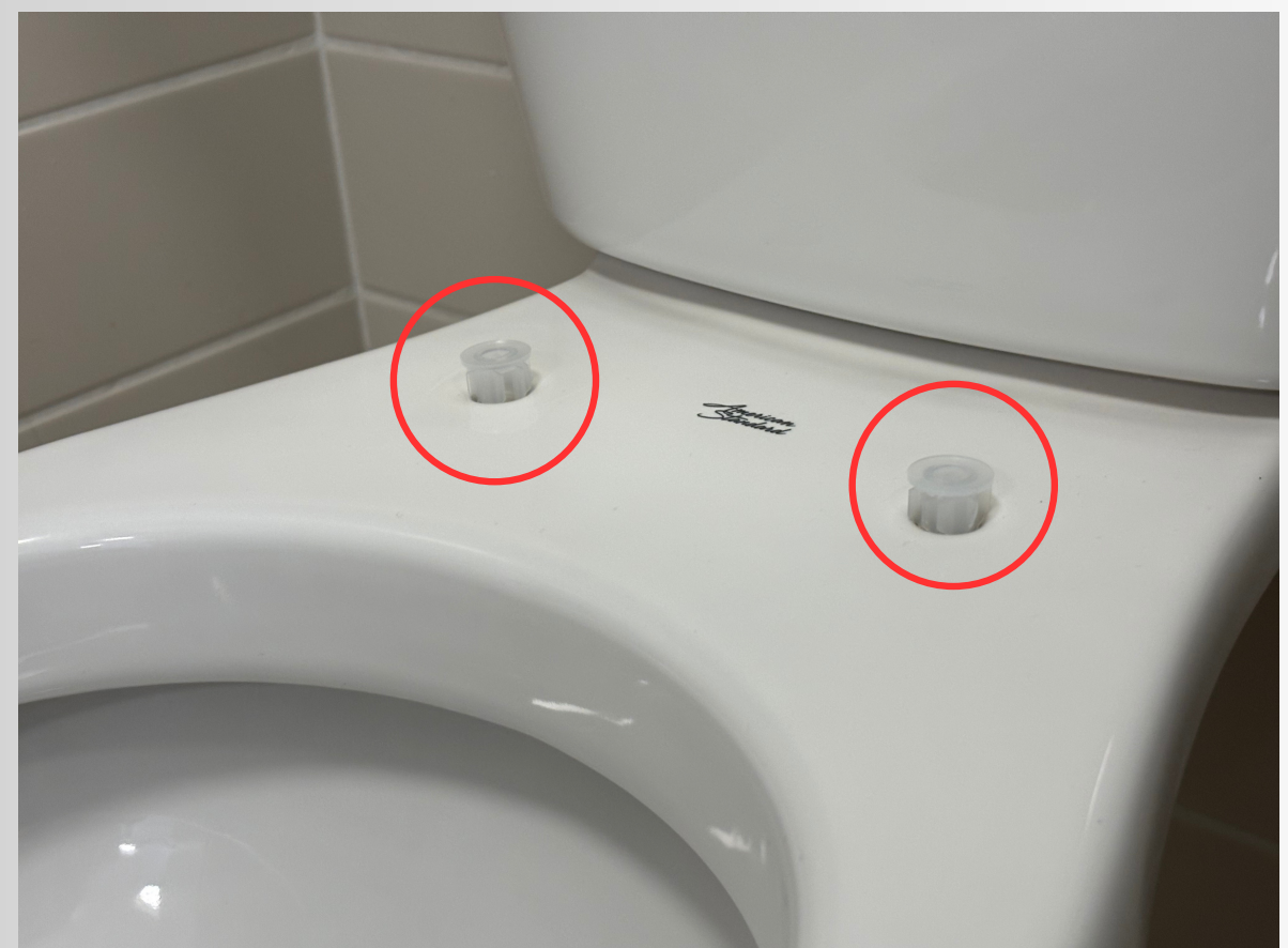
Make Sure the Expansion Plug Is Fully Inserted (Hammer May Be Required).
