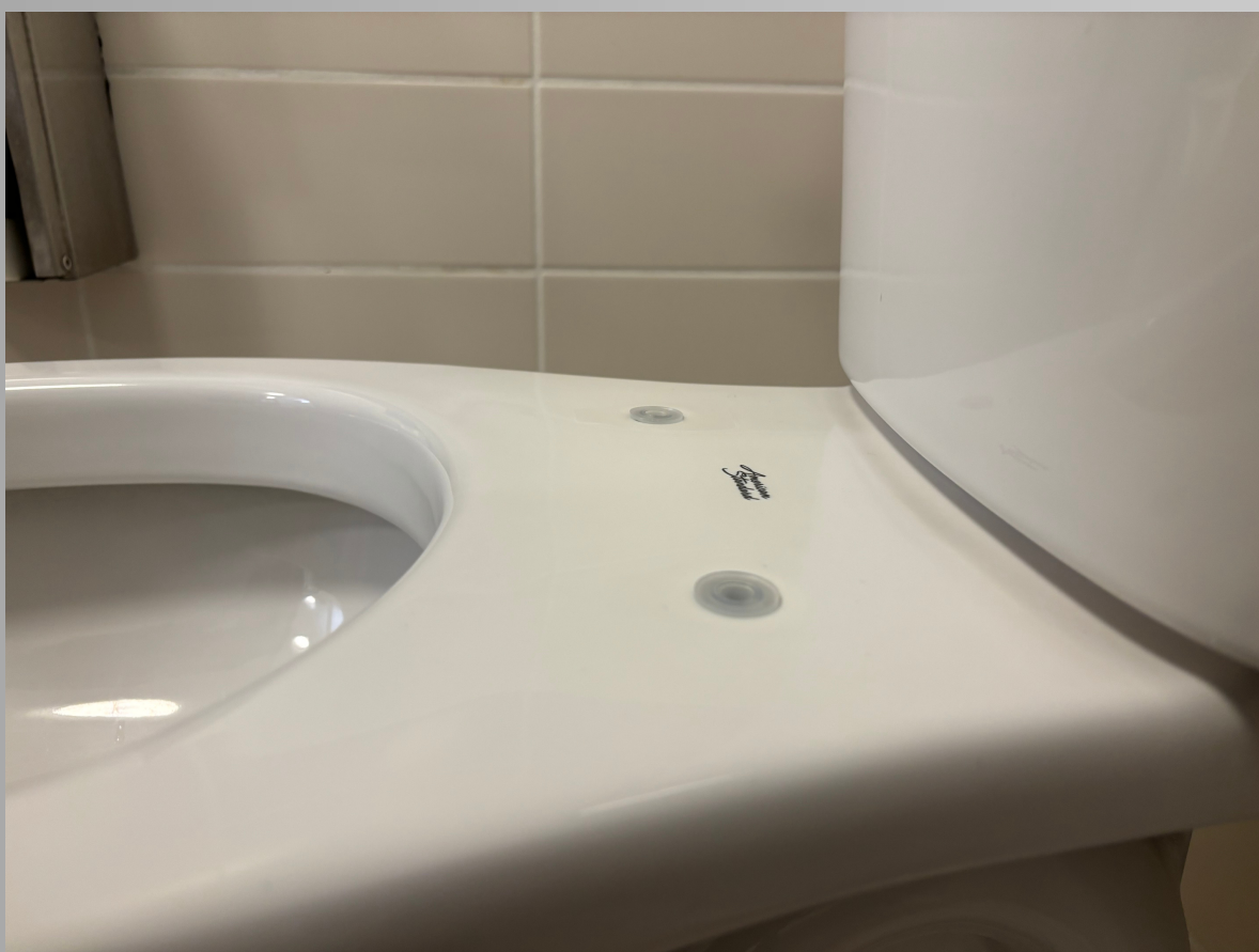
Insert The Expansion Plug To The Installation Holes
