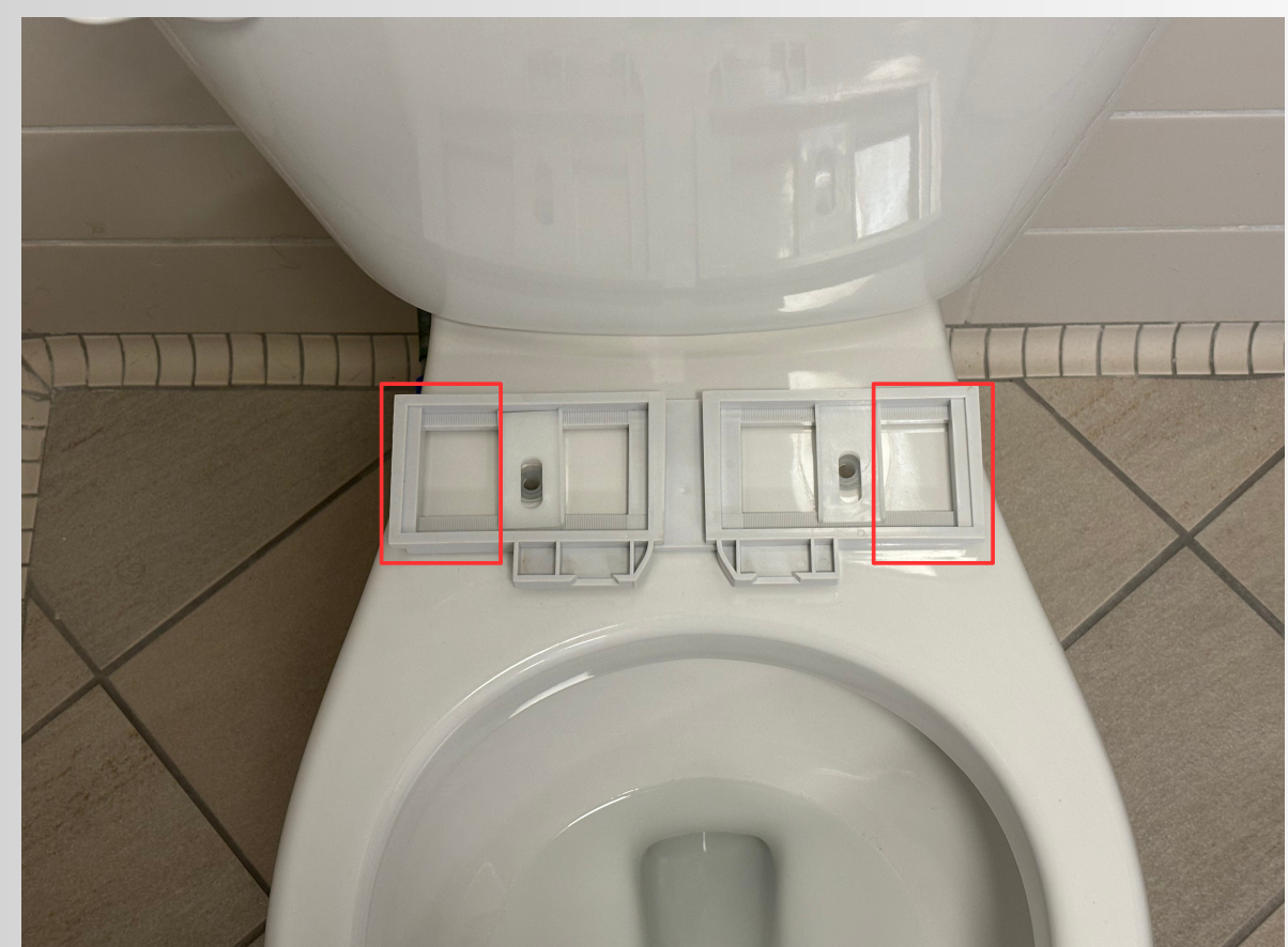
Adjust Mounting Base And Spacers To Suitable Position (Make Sure The Space Are The Same and the Spacers Are Straight )
