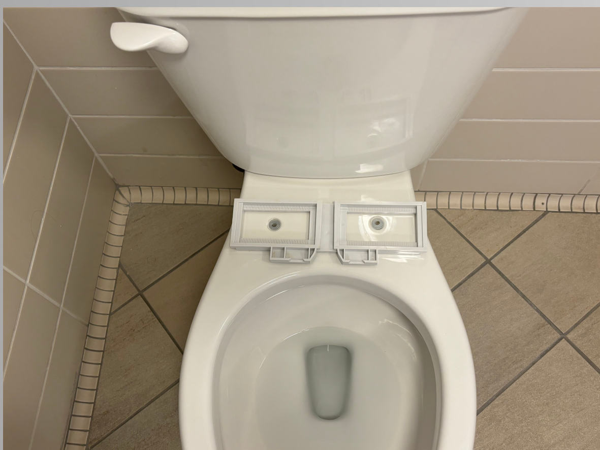
Place The Mounting Base On The Toilet
