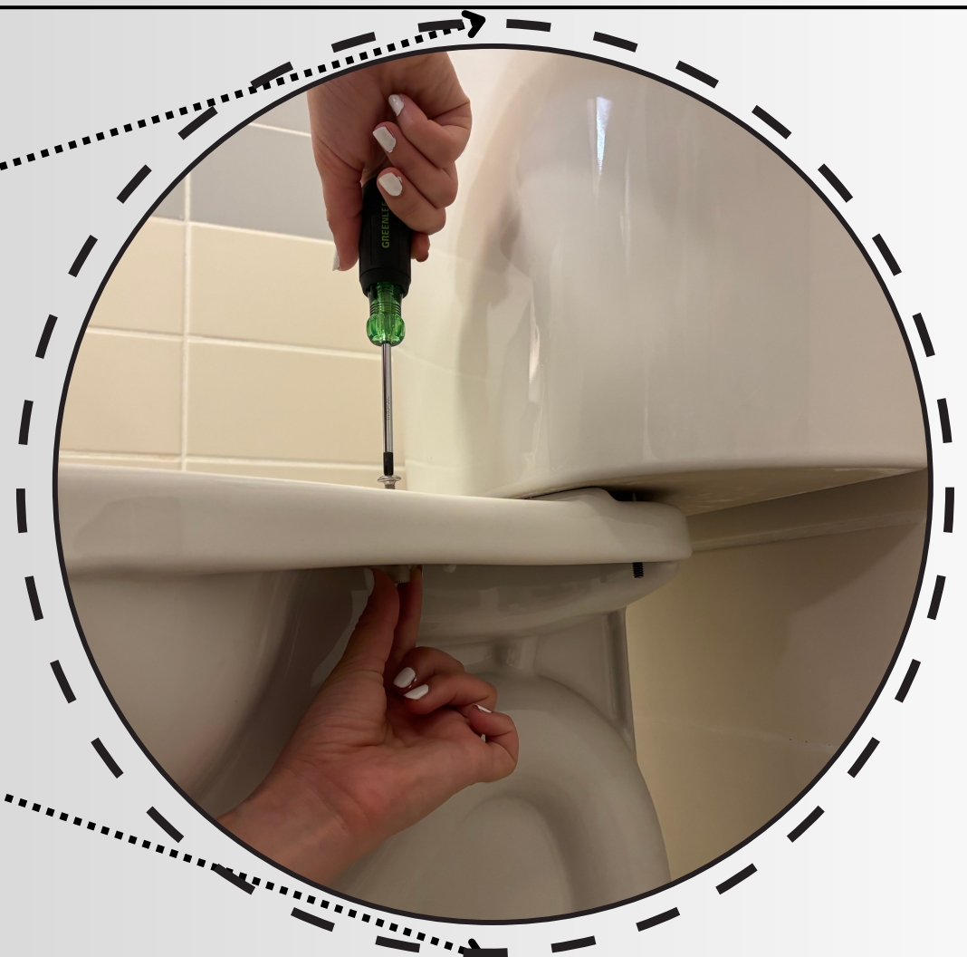
To Tighten The Screws, You Might Need To Hold The Expansion Plug From The Bottom.
