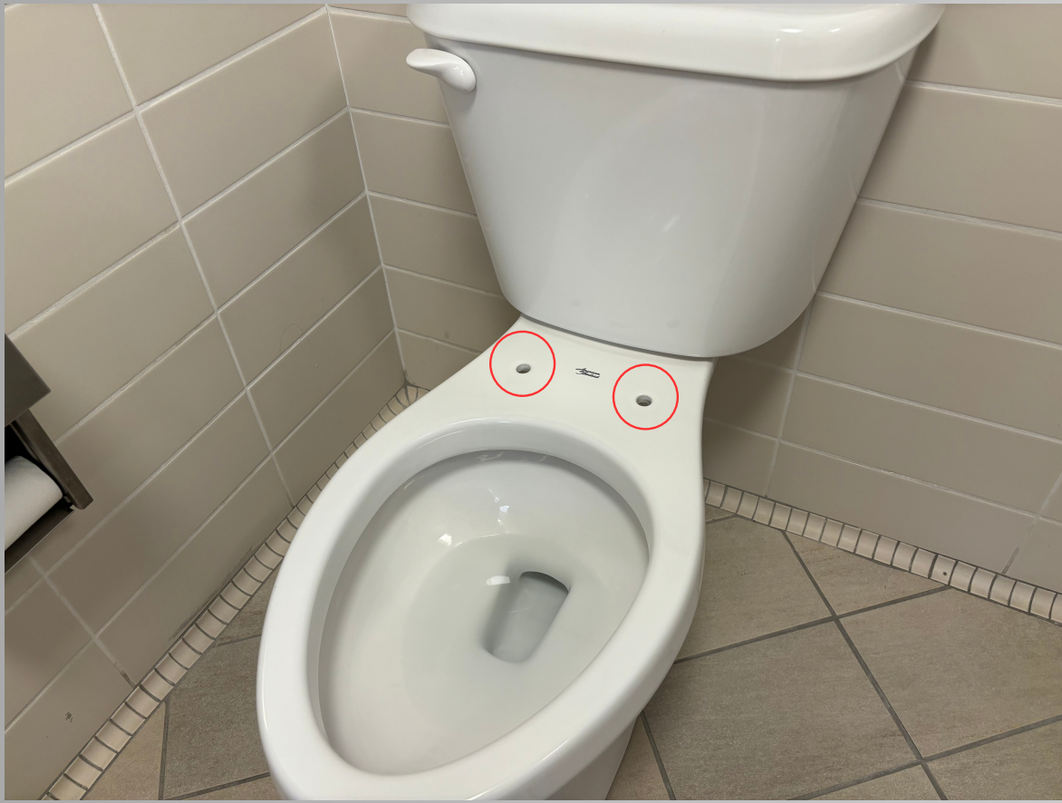
Remove The Original Toilet Cover And Find The Two Holes
